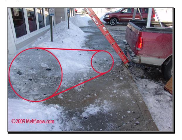
While at first glance this seems like an effective approach, the cost of replacing this section of roof in spring, plus the virtual guarantee of water damage from the now missing roof allowing water to get into the sheathing and eve might be a false economy. Remove the ice dam and replace the roof!
