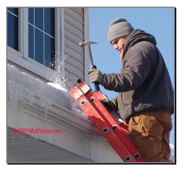
Looks like a good approach eh? Seems that he's effectively chipping away the ice and saving the gutter and roof from water damage inside the building by removing the ice completely...right? Well maybe not.
