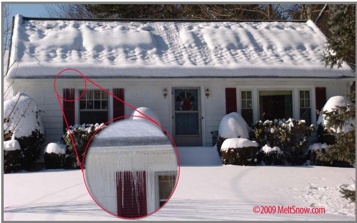
Notice how the rafters of the roof structure are silhouetted by the snowpack on the roof. That's because warm air leaking into the attic space is in turn melting the snowpack on the roof, however the rafters
