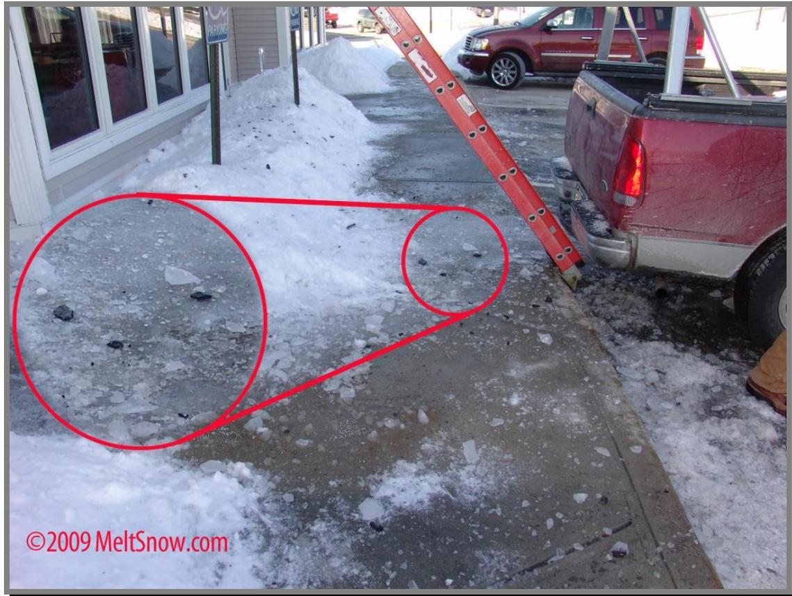
While at first glance this seems like an effective approach, the cost of replacing this section of roof in spring, plus the virtual guarantee of water damage from the now missing roof allowing water to get into the sheathing and eave might be a false economy. Remove the ice dam and replace the roof!
