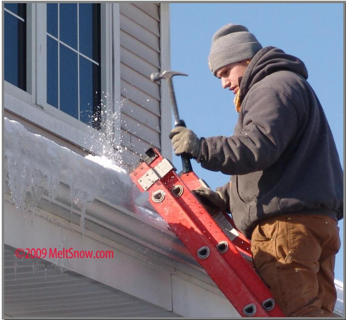
Looks like a good approach eh? Seems that he's effectively chipping away the ice and saving the gutter and roof from water damage inside the building by removing the ice completely...right? Well maybe not.
